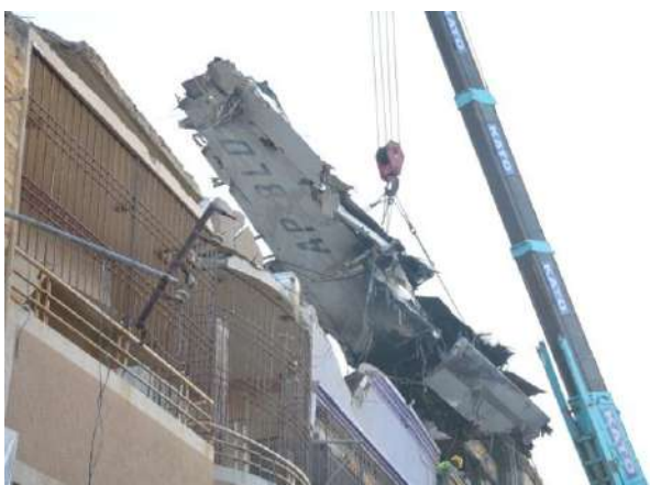
Fig 7 : Left wing being lifted from roof top
